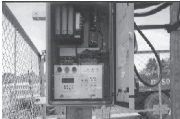
Fig. 6.3: Control unit for auto-recloser
