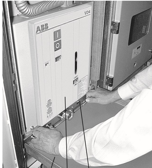
Figure 4/4: Service truck engaged with the panel. Withdrawable circuit-breaker part released for removal by moving the sliding handles inwards
