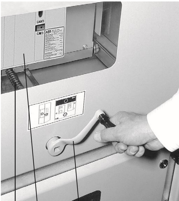
Figure 4/2: Movement of the withdrawable breaker part between the test/disconnected position and the service position, clockwise up to the stop for the service position and anti-clockwise for the test/disconnected position
